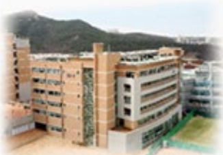
Whole view of GSPA Bldg. 57-1
